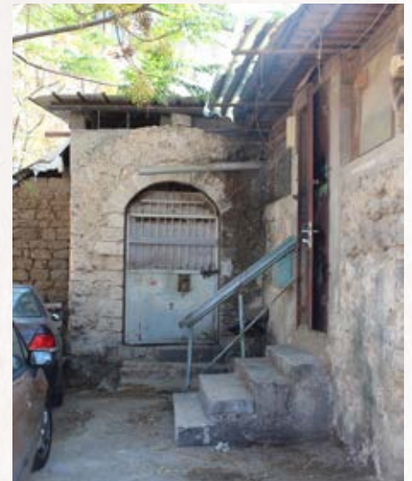
One of the original Batei Varsha buildings.
