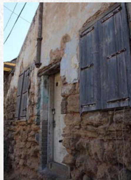
One of the original Batei Varsha buildings.
